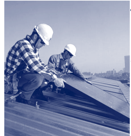
Workers install solar panels on the roof of the Olympic aquatic center in Atlanta.
